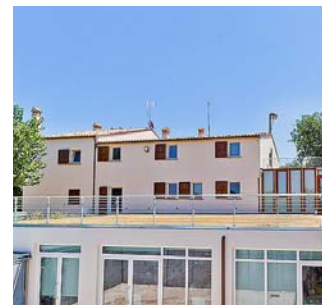
PROVINCE OF PESARO (ITALY) ENERGY EFFICIENCY: MECHANICAL, ELECTRIC AND SPECIAL PLANTS
